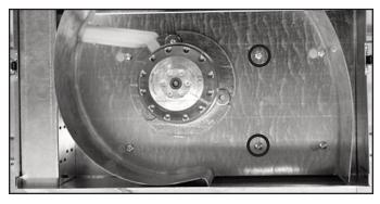
Align damper screw holes with holes in hood to properly position the damper on hood. Using two (2) standard  $\frac{1}{2}$ " screws (1 per side), secure the adapter to the top (or back) of the hood). Seal the adapter to the hood using duct tape.
