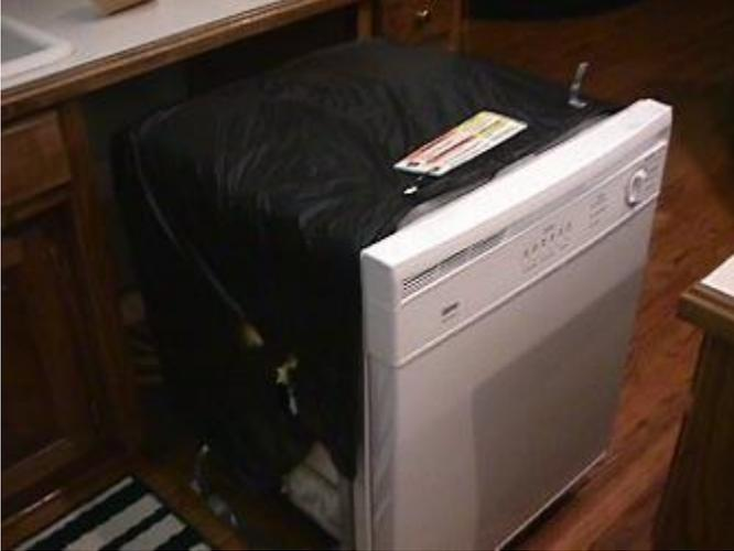
**Step 6. Gently push the appliance back into the cabinet, bend the bracket back to the underside of the counter and reinstall the two holding screws. You' are now ready for peace and quiet.**
