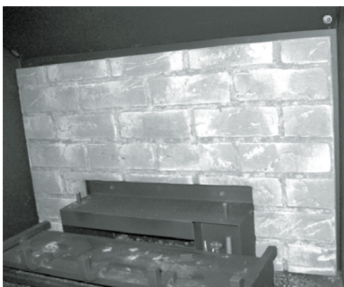
Back Panel Installed
