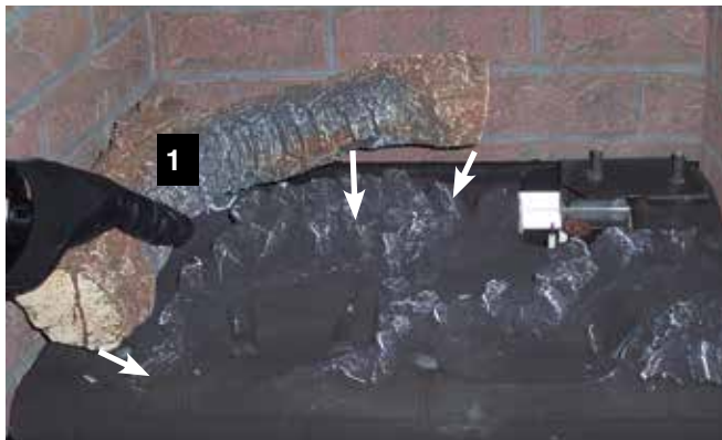
Log 1 location on burner
