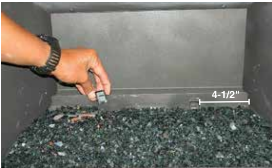
Log bracket install
