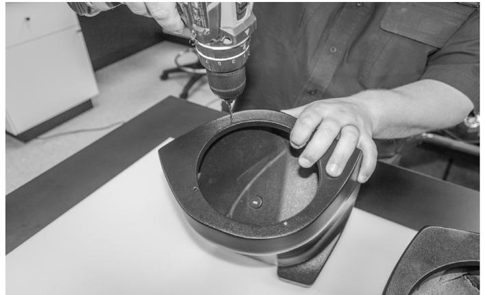
Next prep the speaker pods by drilling the holes in pods. The pods come with the mounting hole locations already marked. Use 1/8" bit to clean out the holes to prevent damaging the screws or enclosures.
