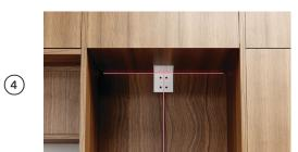
Measure the height from floor to the front overhang and mark on rear wall.
