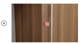
Using a piece of tape, fit a tab on the door to assist in opening the door without disturbing panel settings.
