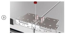
Secure the bracket at the front top using four screws.
