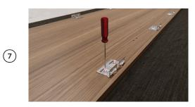
Secure the side brackets using two screws per bracket. Ensure side brackets are fitted tightly and the fasteners are secured straight.
