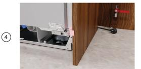
Push product into alcove while pulling the hose and power cord. Ensure the gauges touch the alcove end, the hose doesn't kink and the power cord remains free and untangled.
