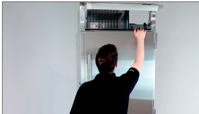
FIG. 3. Be sure to inspect behind the rainshield.
