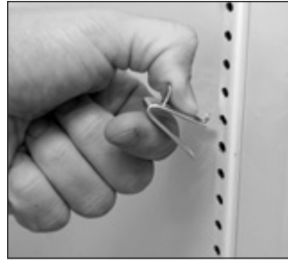
FIG. 1. Installing top tab of shelf clip.
